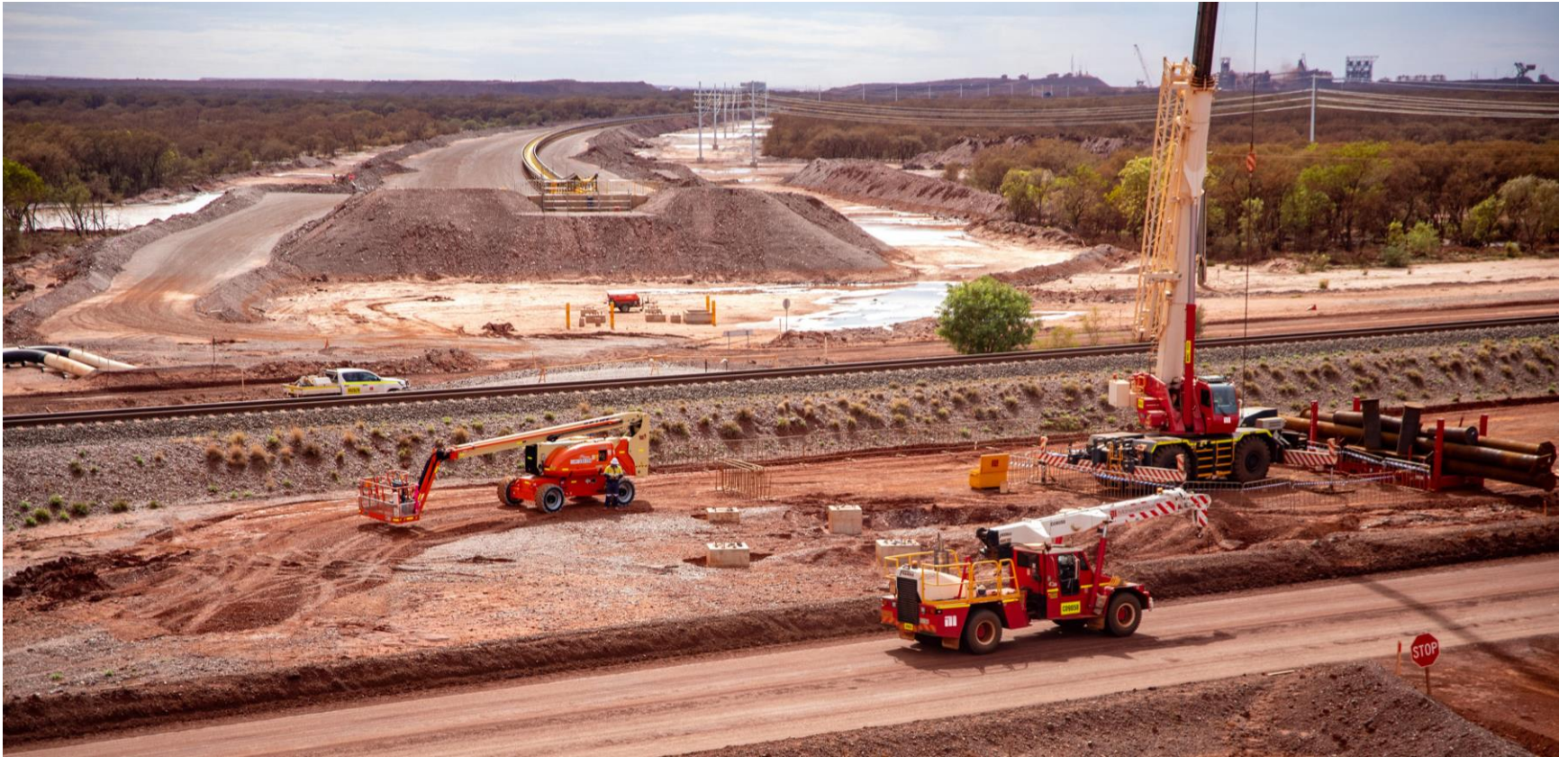
Construction of Fortescue's Christmas Creek overland conveyor, Pilbara region, Western Australia.
