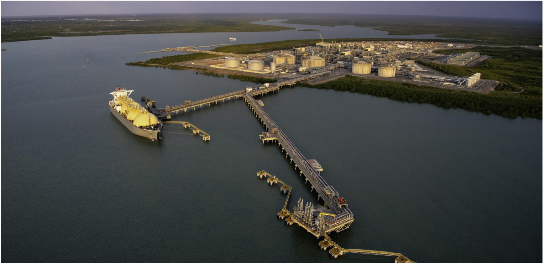
INPEX-operated Ichthys LNG onshore processing facilities, Bladin Point, Darwin, Northern Territory.
