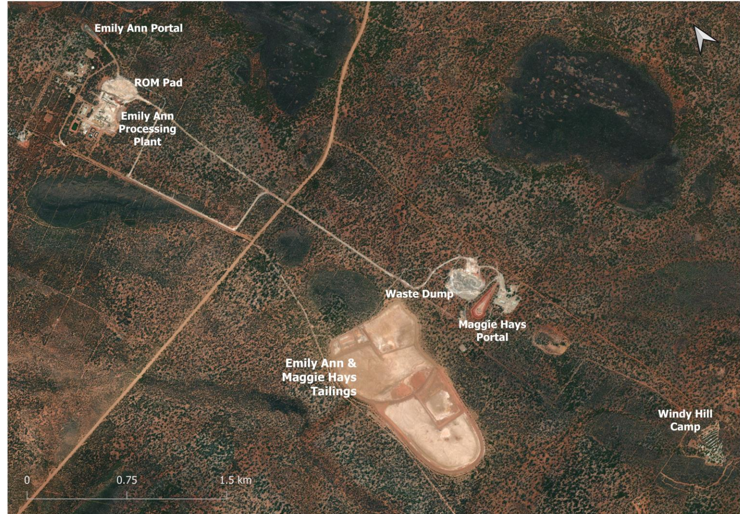
Lake Johnston – Significant Infrastructure
