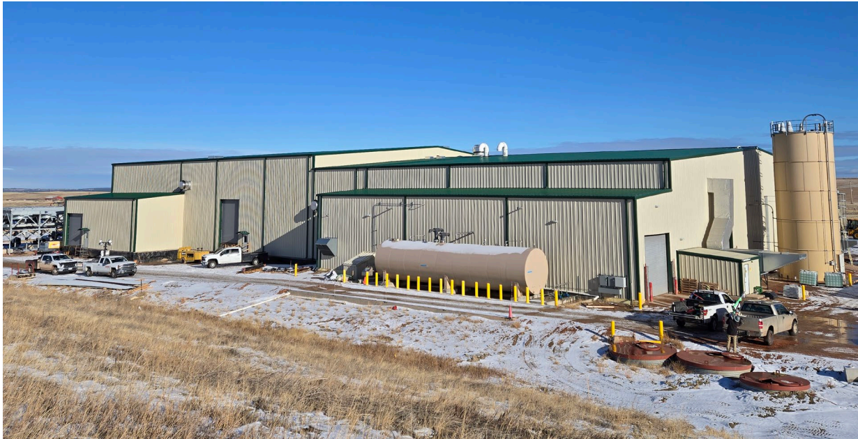
Figure 1: Peninsula Energy's Lance Central Processing Plant, December 2024
