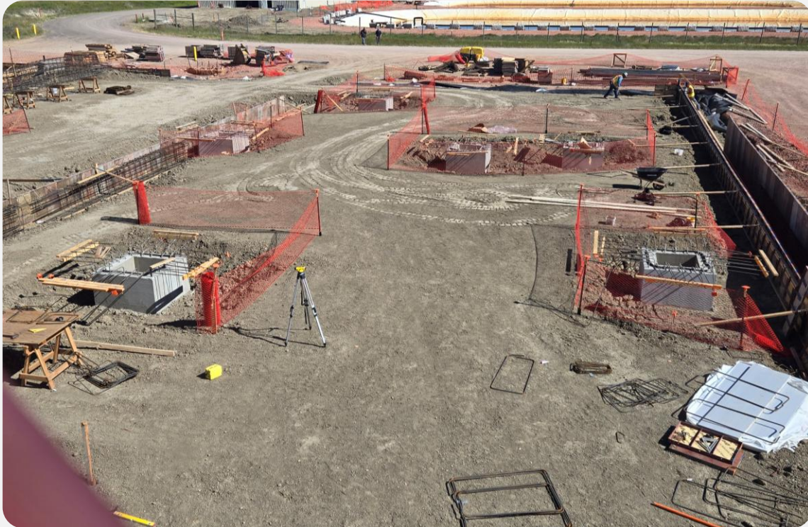
Lance Central Processing Plant Site: Early July 2024
