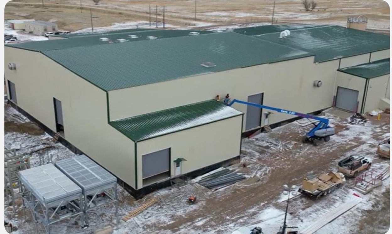
Lance Central Processing Plant: Early November 2024
