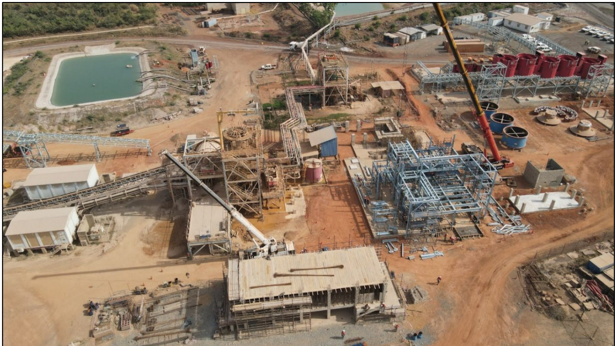
Figure 3: The milling area substation is 15% complete
