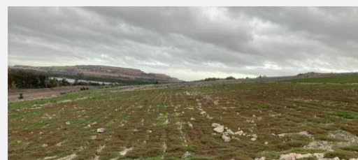
Peak Downs Rehabilitation Works
