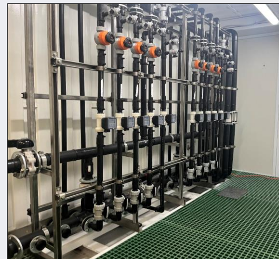
Wellhouse Module (pipe room)
