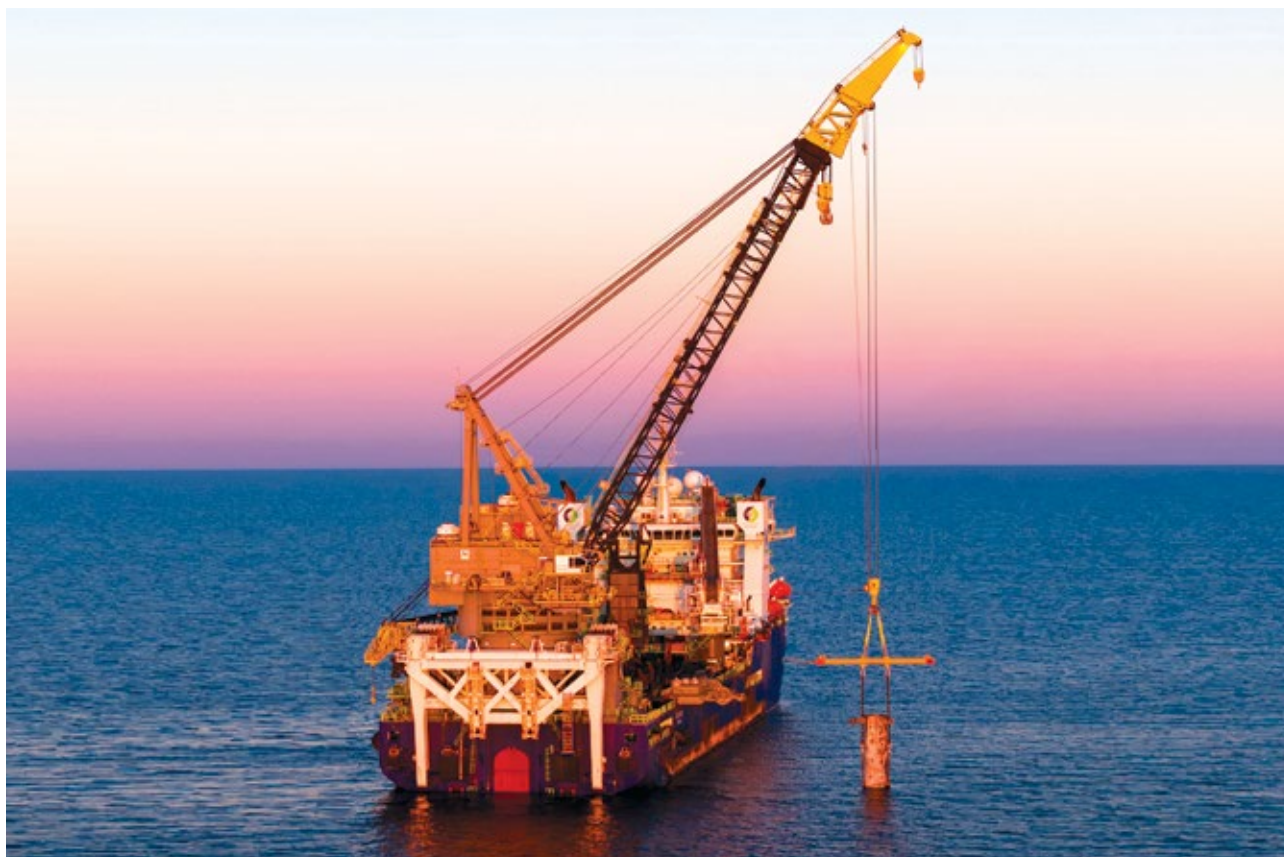
Pictured: Campbell Decommissioning Project
