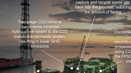
Thermal oxidiser reduces the amount of methane emissions by oxidising the methane before release
