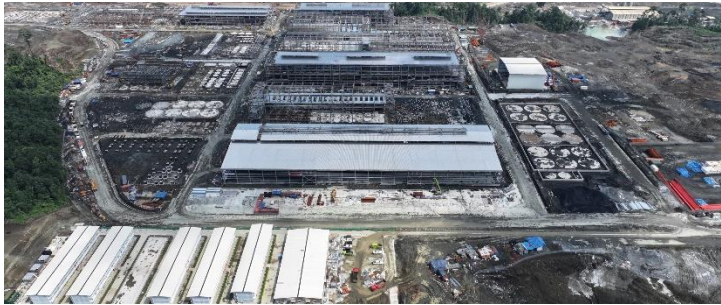
ENC HPAL, sulphate and cathode plants ahead of schedule
