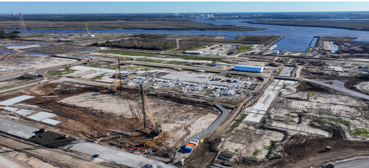
Woodside Louisiana LNG development, January 2025
