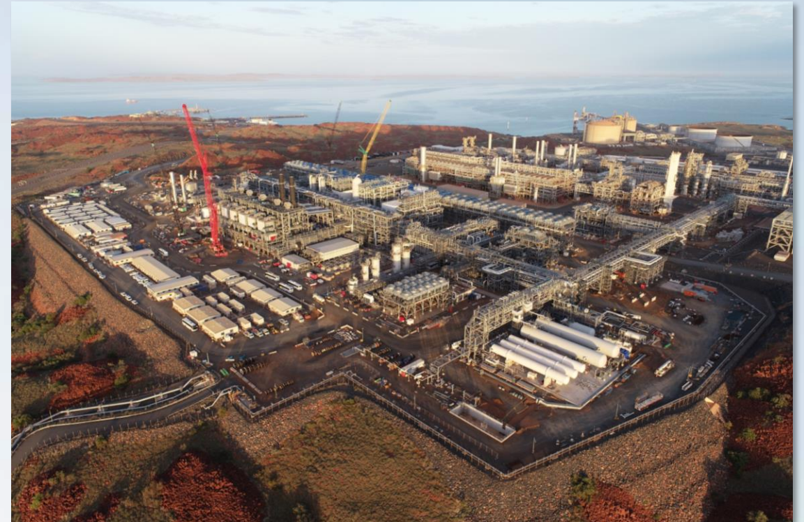
Pluto Train 2 construction progress
