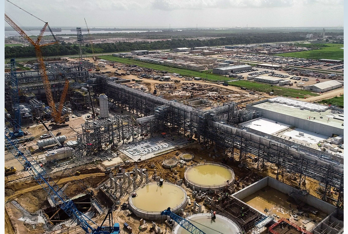
Beaumont New Ammonia Project under construction
