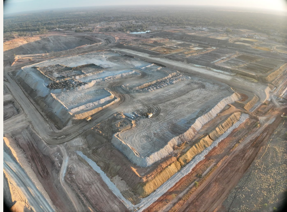
Progressive mine rehabilitation of old heap leach pads underway using clean waste rock from Murrawombie Pit
