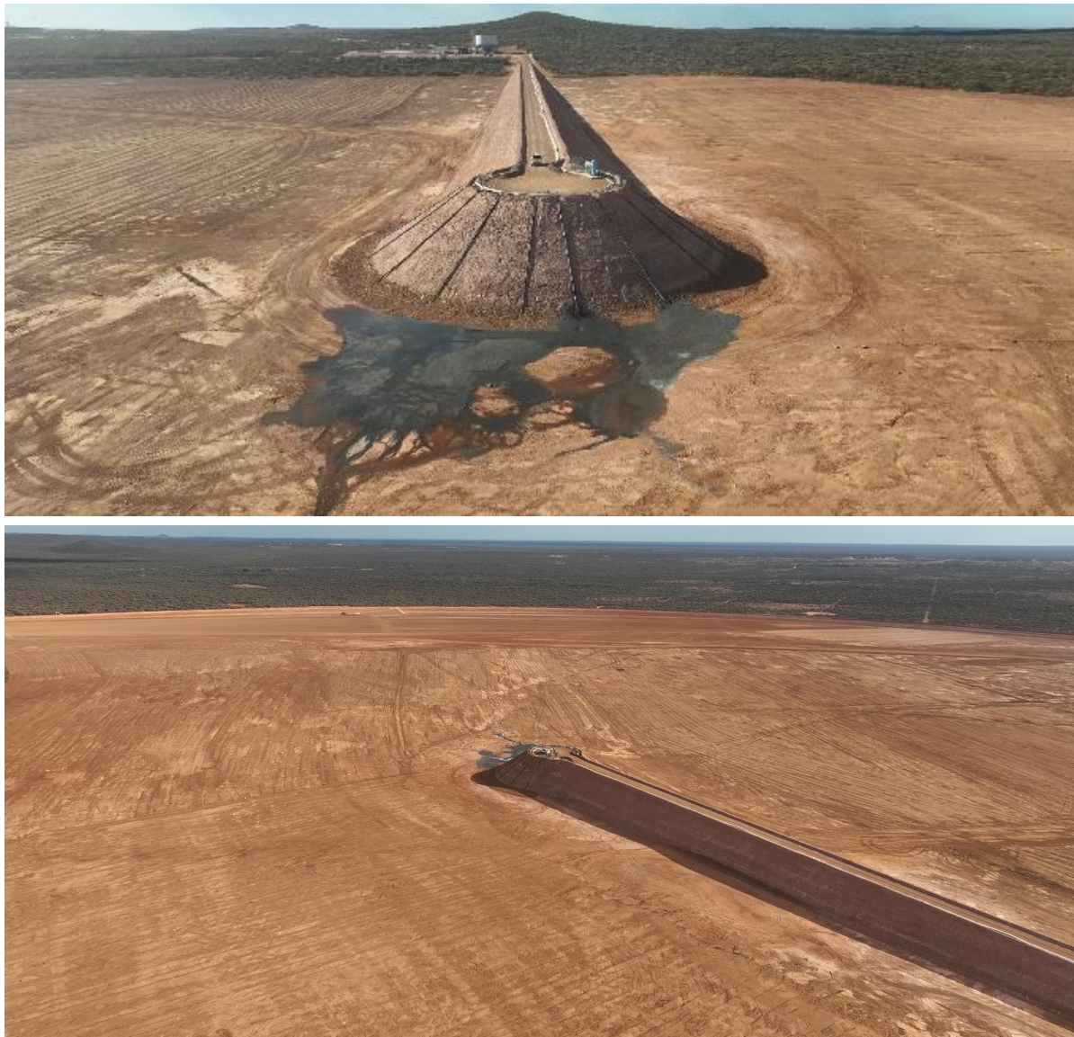
Figure 4: Deposition of tailings at TSF 4
