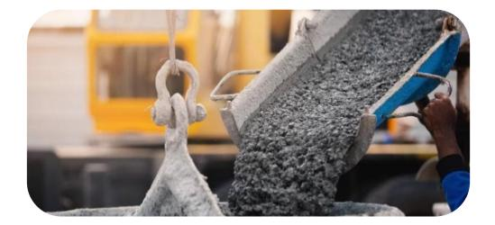
Addition of 1 kg of Great White HRM<sup>™</sup> per m<sup>3</sup> in standard concrete mixes lowers the required water and cement by ~8%
