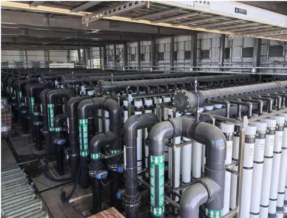
Ultrafiltration installed
