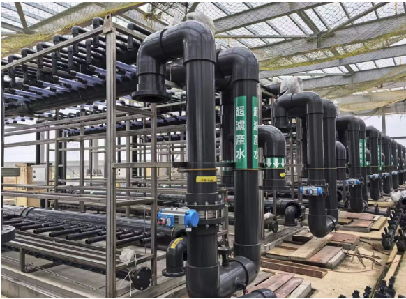
Ultrafiltration-Installation
