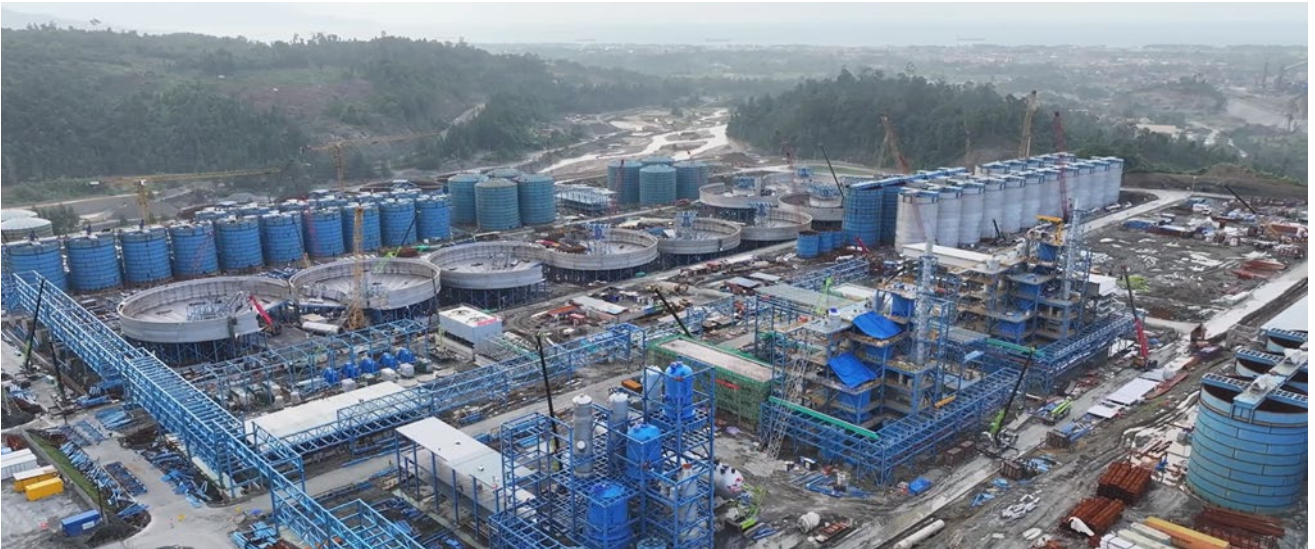
Autoclaves, including pre- and post-treatments shown in the foreground
