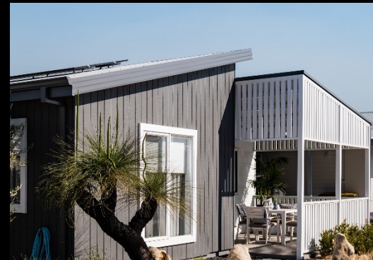
Housing Piara Waters WA
