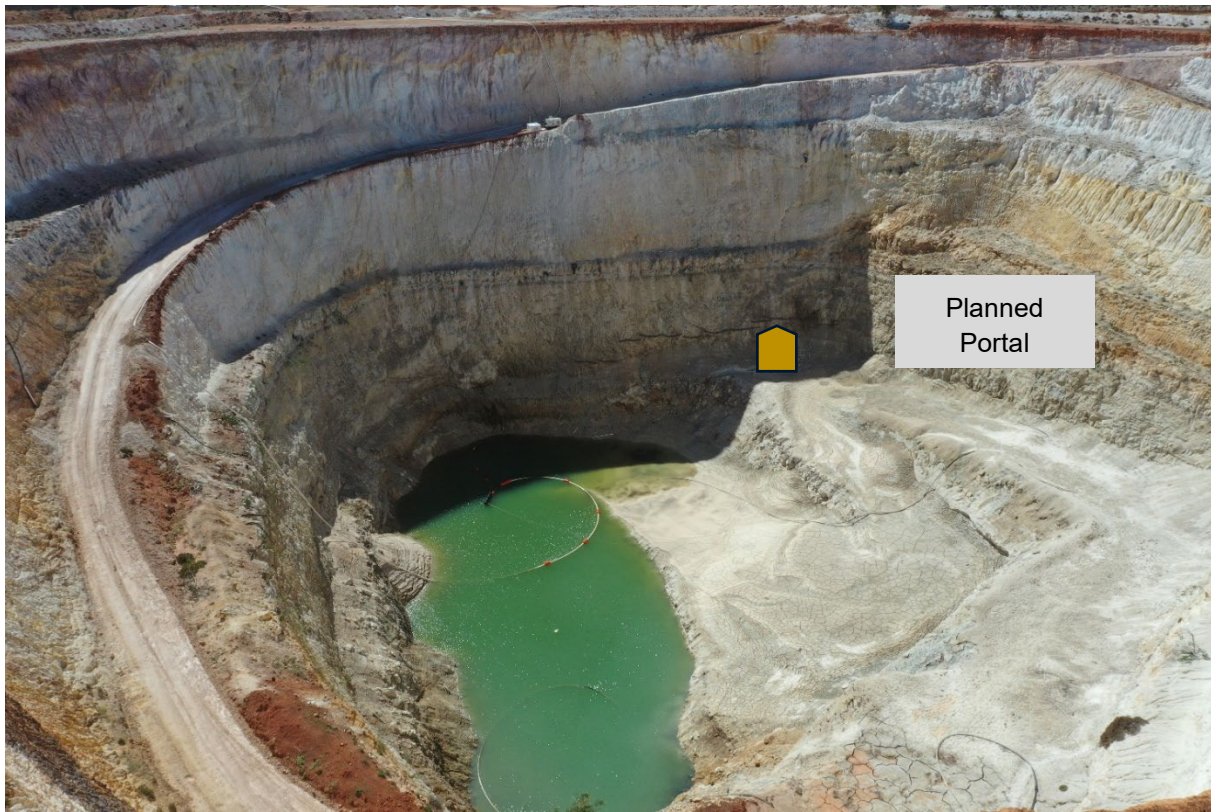
Figure 1 – United North pit showing planned decline location and completed meshing
