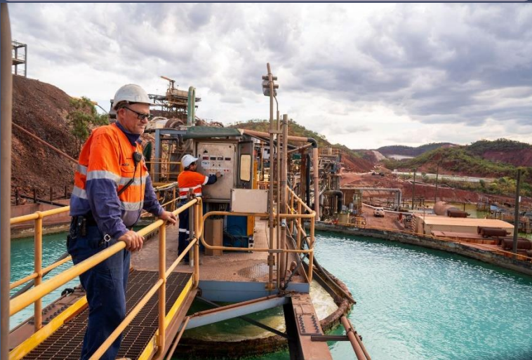
Processing plant & surface infrastructure
