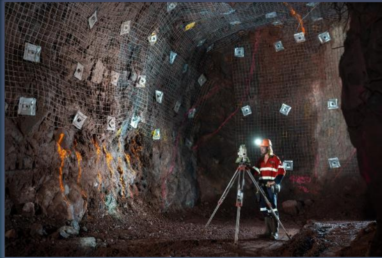
Established underground development
