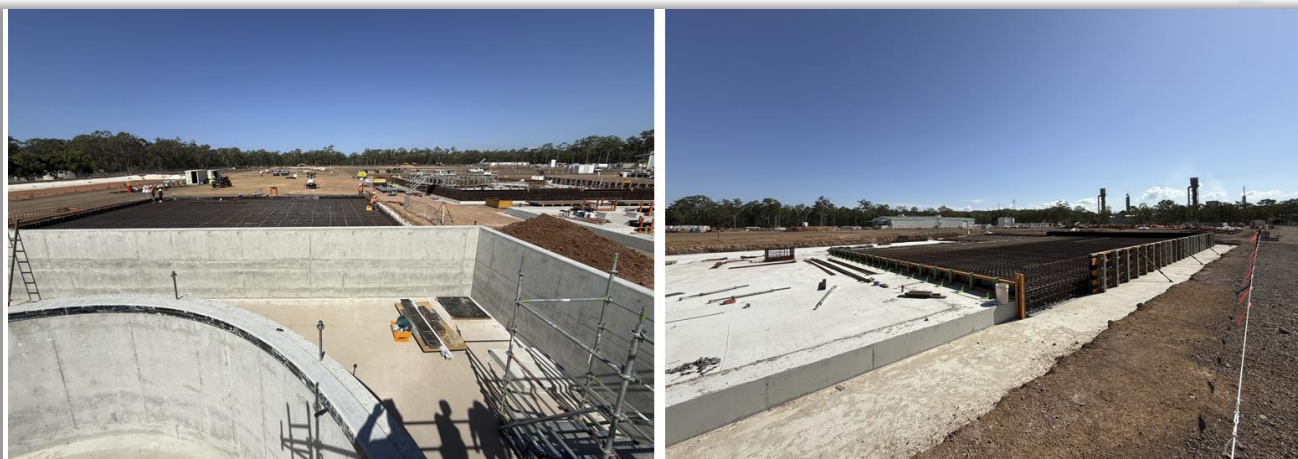
Orica Reagent Storage and SX foundation steel work
