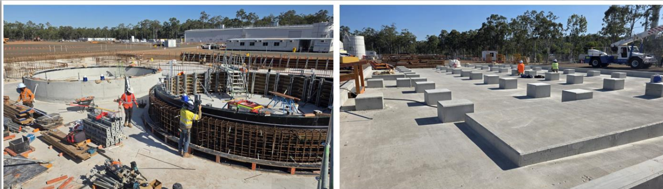
By-Product and Evaporator foundations in construction
