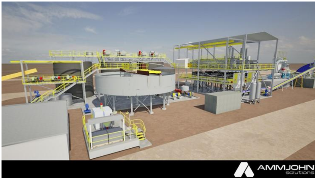
Figure 3 - Stage 1A+ Dewatering Area, showing Thickener and Filter Press
