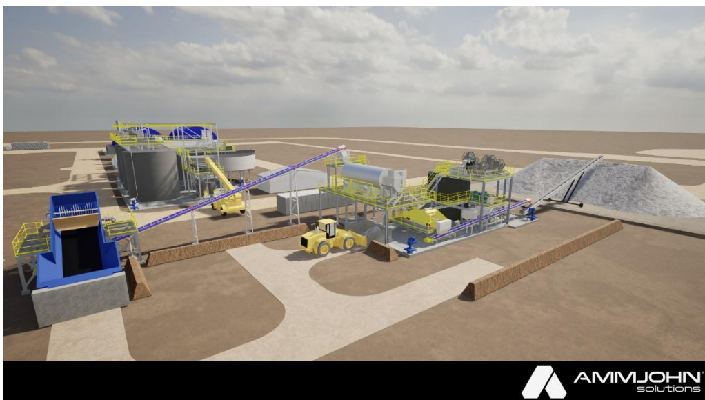
Figure 2 - Stage 1A+ Blundging area showing Drum Washer and Hydro-cyclones
