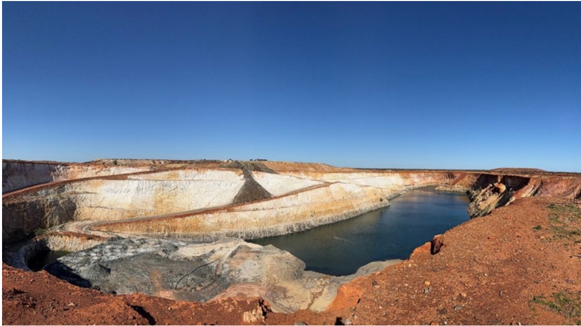
Figure 3 – Youanmi Main pit pump showing a ~9m reduction in water level
