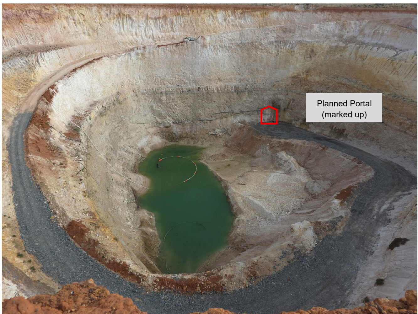
Figure 1 – United North pit, road repaired, face meshed and Decline marked up
