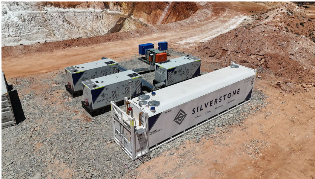
Figure 2 – United North Power Station progressing to commissioning
