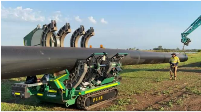
Rising main pipeline being extended to the next stage, June 2025.
