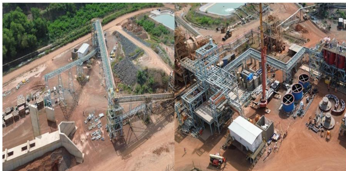
Figure 2: Secondary Crushing and Ball Mill Areas
