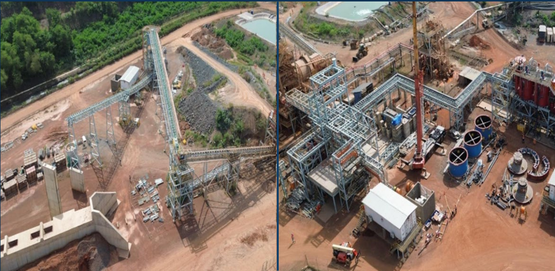
Secondary Crusher circuit and Ball Mill areas
