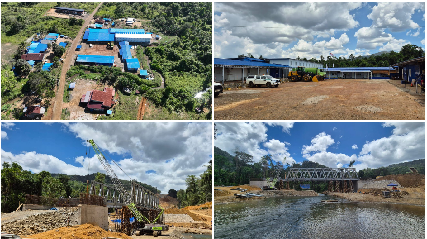
Sampala Mine camp and bridge construction
