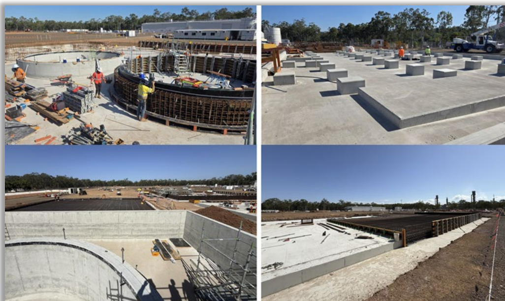
Site civils and concrete activity
