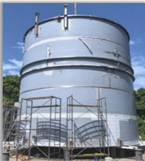
Completing trial assembly of large volume reagent and by-product tanks
