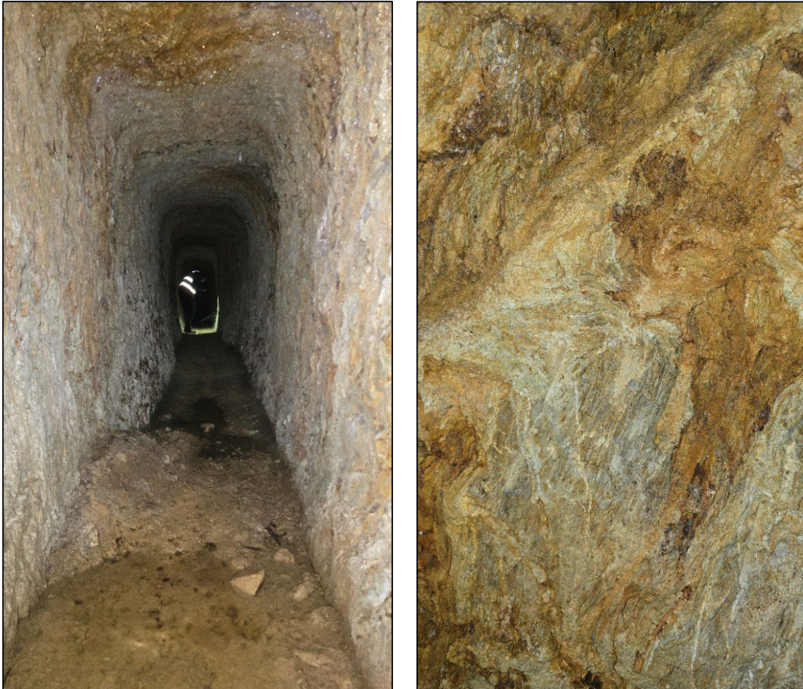
Figure 3: Previously undiscovered adit at Coupon Prospect exposing a west dipping strong altered reverse fault zone (MGA94 Zone 55; 376,013mE; 5,333,824mN).
