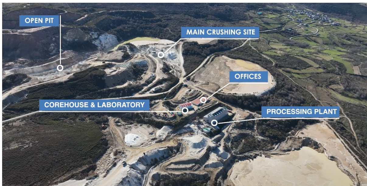
Figure 2: Locations of facilities at the Penouta Mine.
