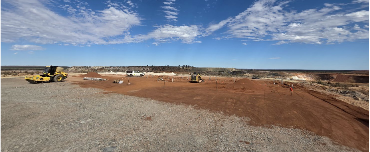
Figure 3 – Preparation for site offices and workshops advancing
