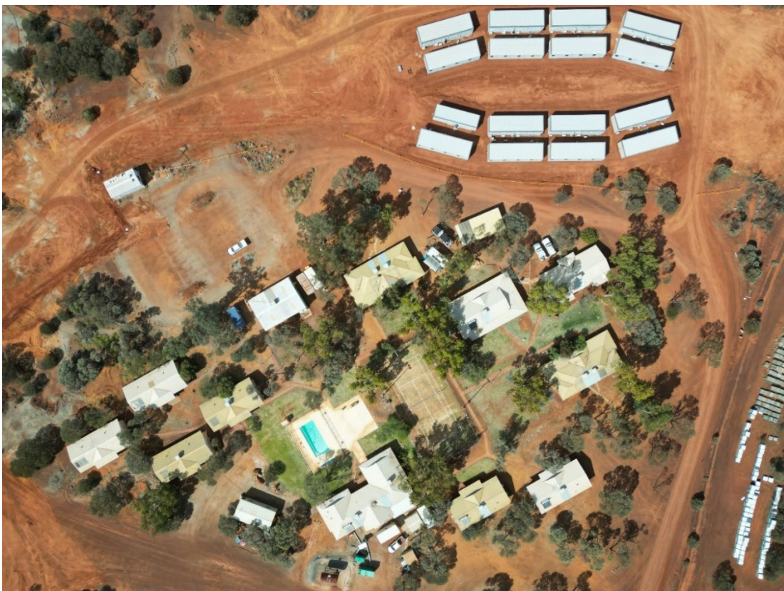
Figure 4 – Phase One Camp Expansion works advancing
