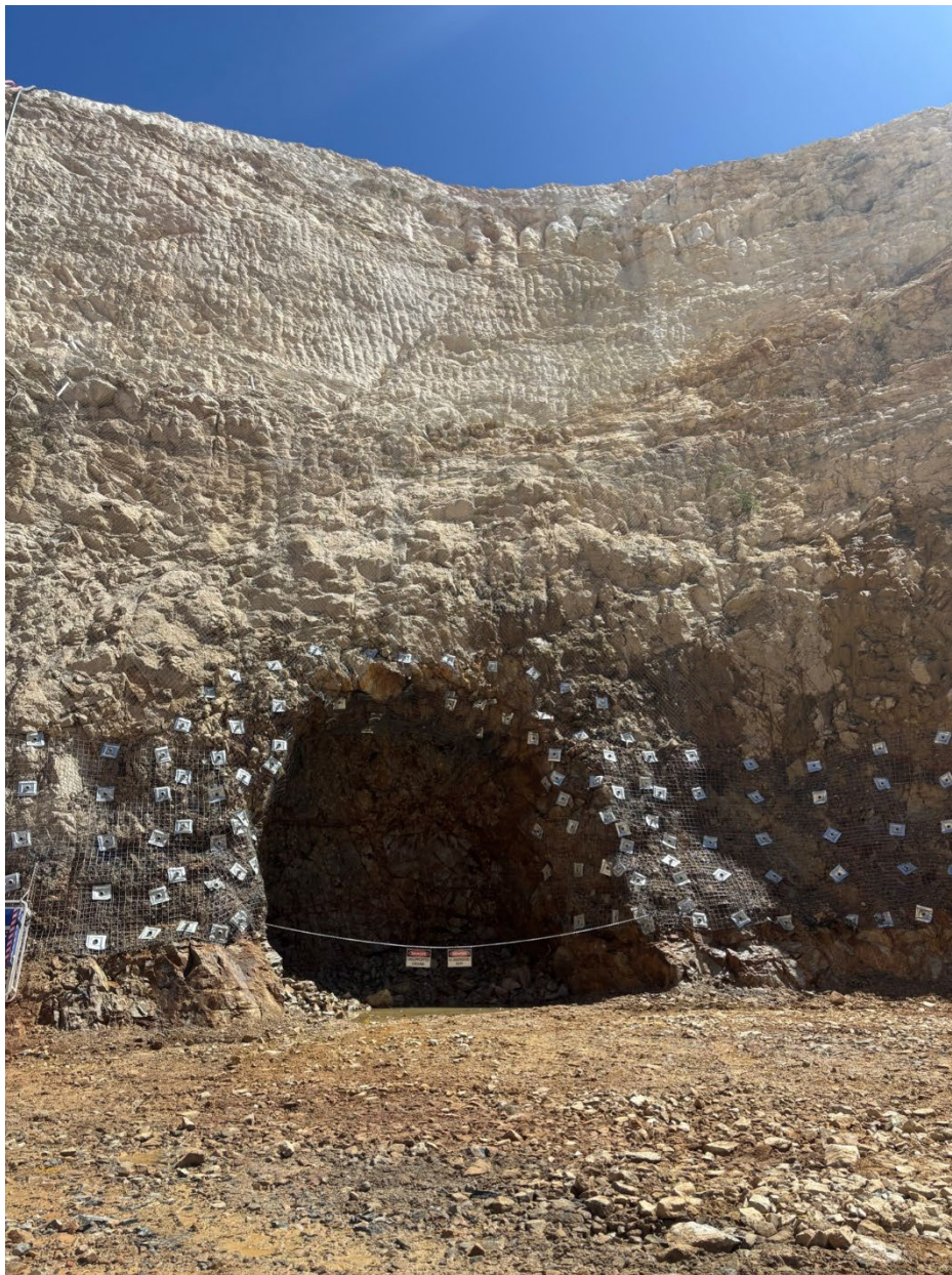
Figure 3 – First cut supported
