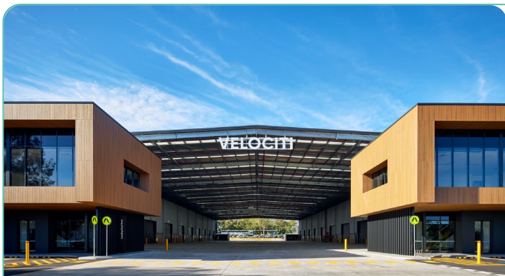
12 Church Road, Velociti at Moorebank (Spec)
