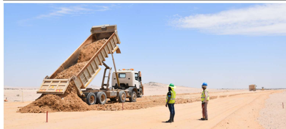
Wide haul road constructed with 100 mm gypsum running board
