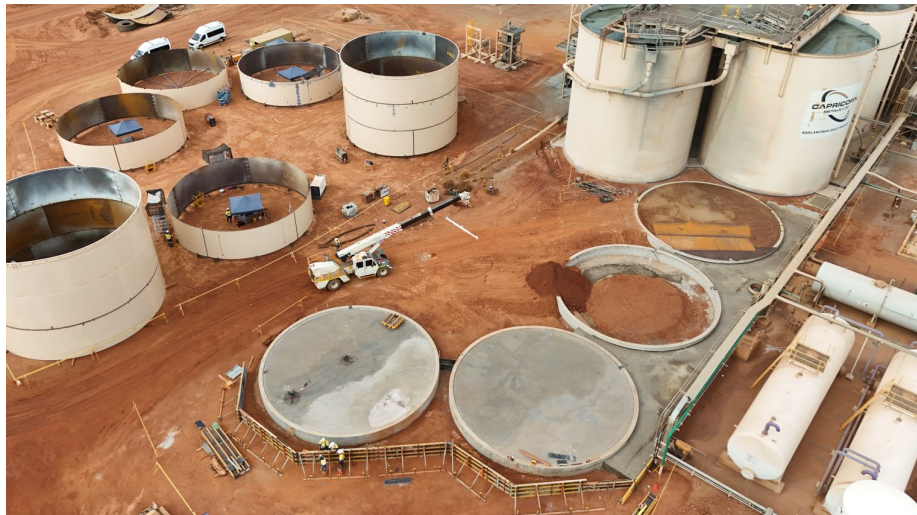
2.) CIL Tank Construction
