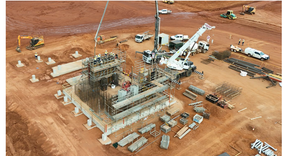
1.) Mill Slab and Feed Trunnion
