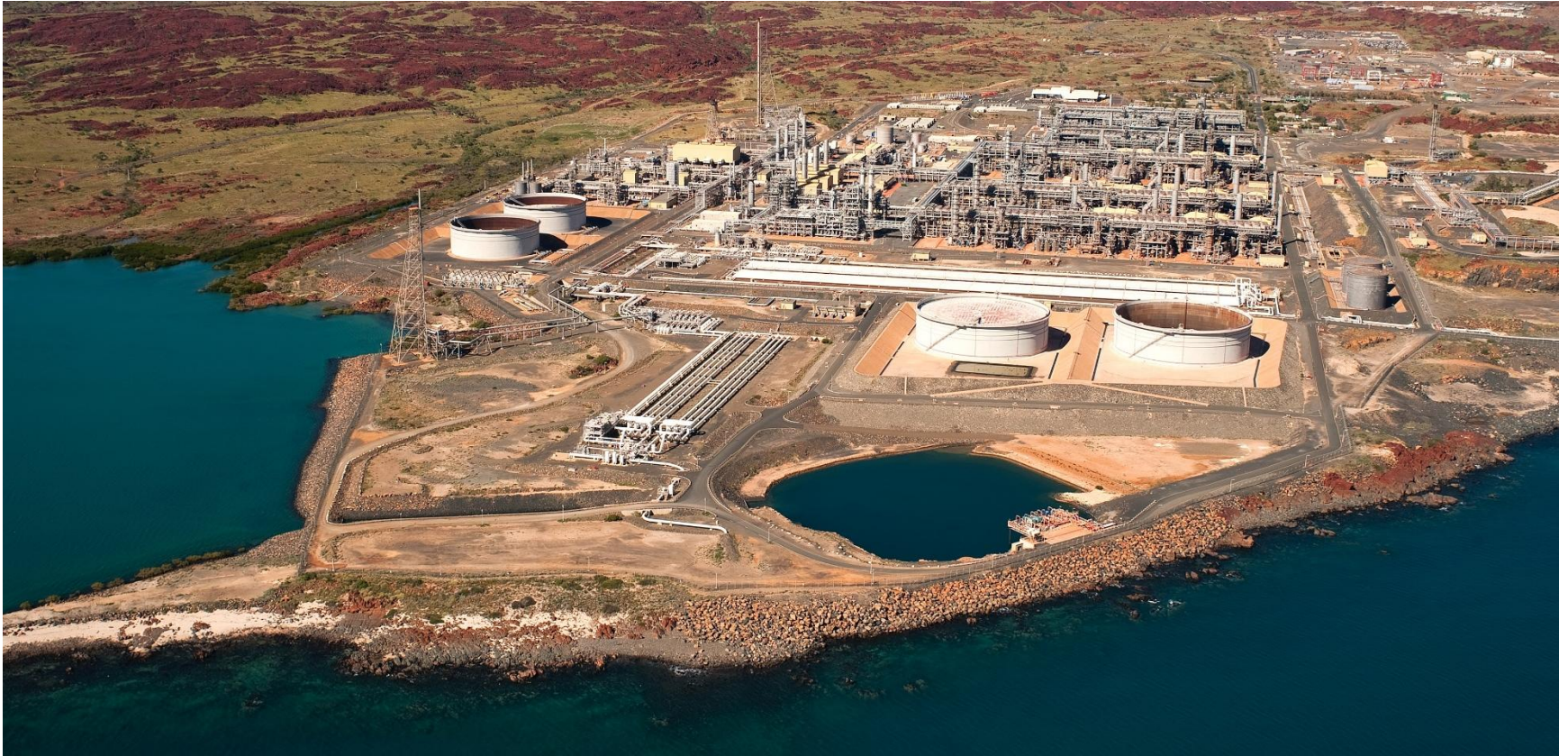
Woodside's Karratha Gas Plant in Western Australia.
