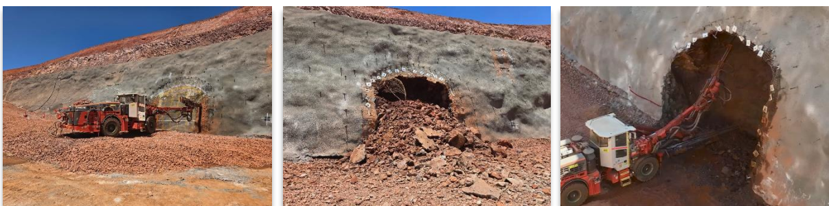
Figure 6: First cut of the Gossan Valley portal
