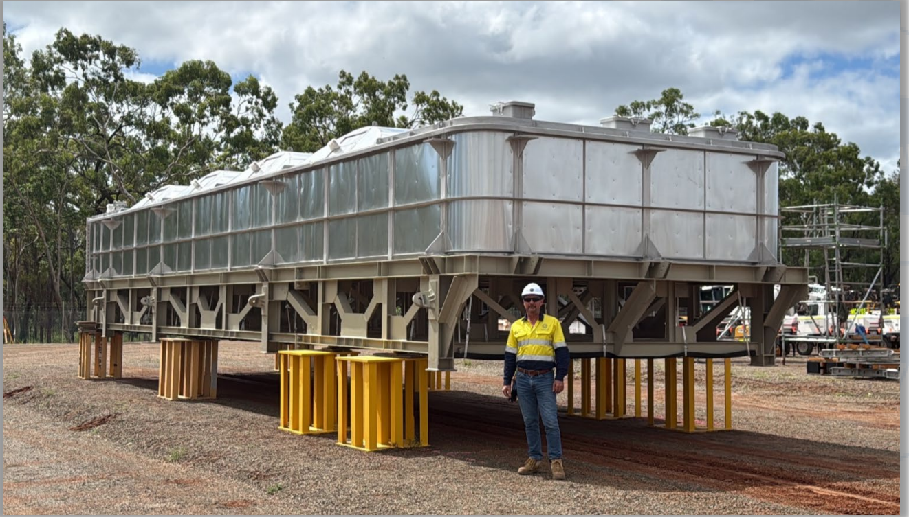
SX Settlers being staged at site for SMP installation – January 2026
