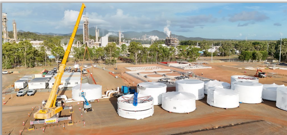
Orica Reagent Tanks staged for installation – January 2026
