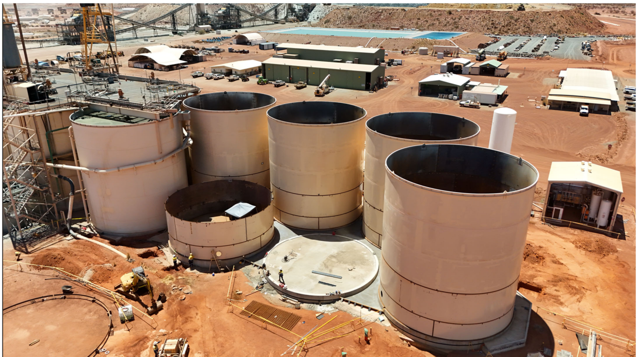
Karlawinda Expansion Project – CIL tank welding and erection.
