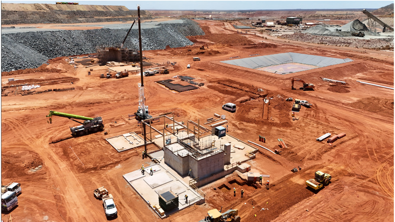
Karlawinda Expansion Project – Major concrete and structural steel works progressed. Mill (foreground) and crusher and ROM 2 (background).
