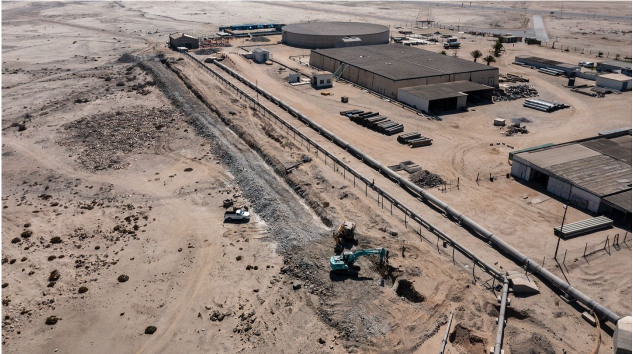
Figure 5: Excavations for the permanent water pipeline have commenced and are progressing in line with schedule.
