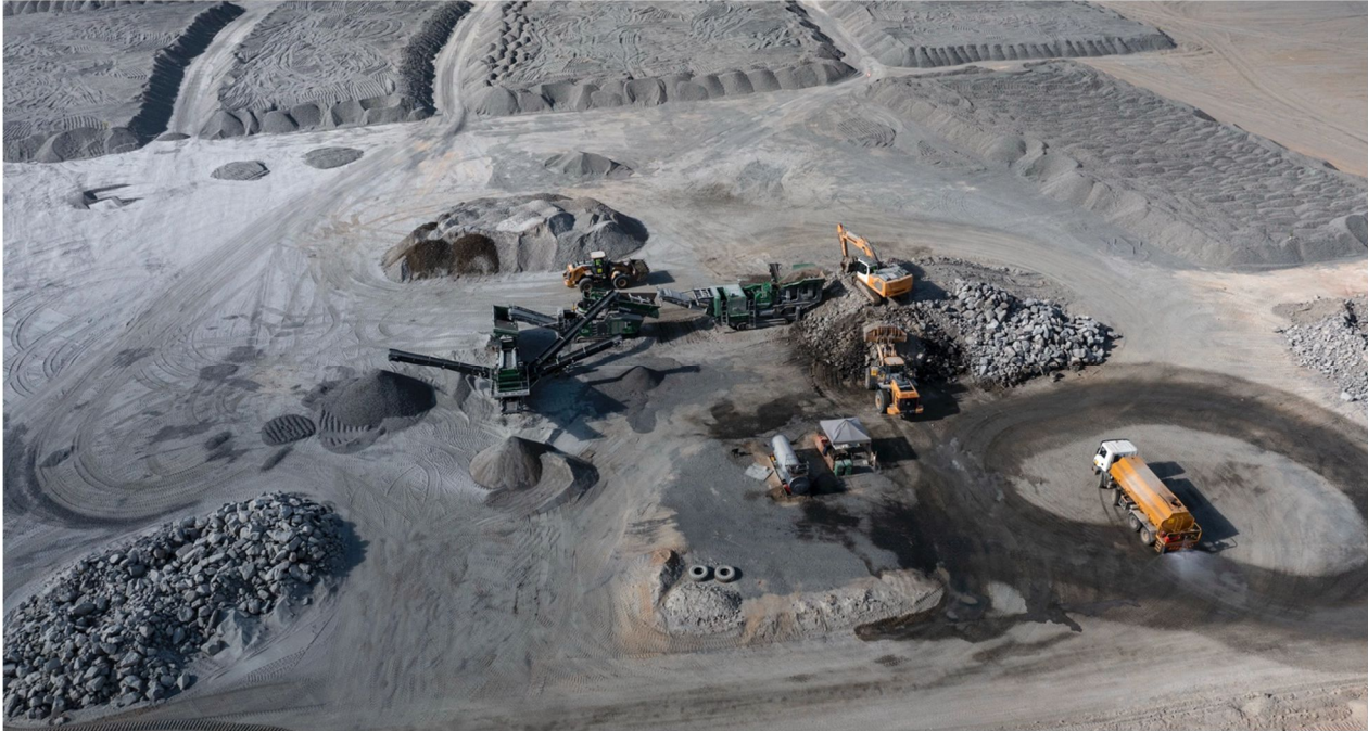
Figure 2: Blasting, crushing and screening of the heap leach drainage material.
