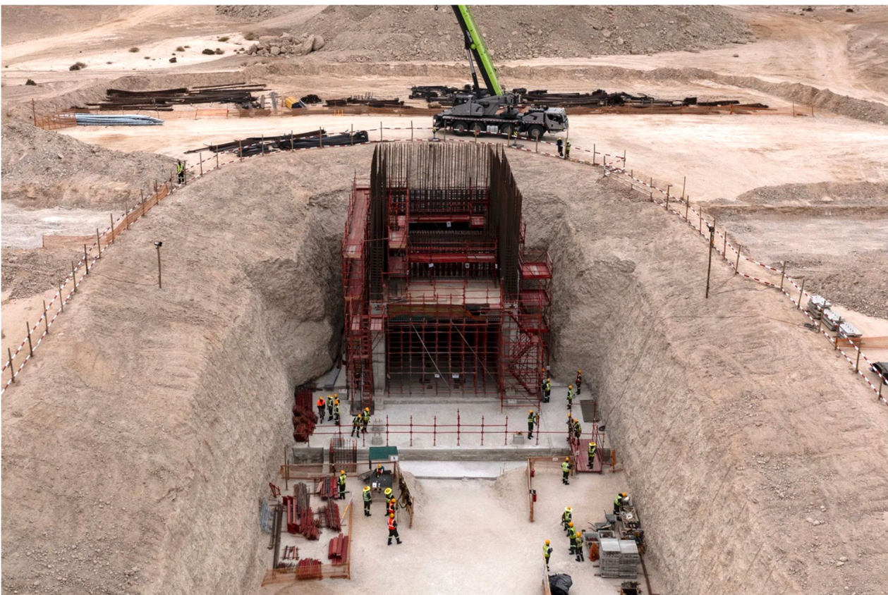
Figure 4: The primary crusher building foundations are complete with the first level walls complete.
