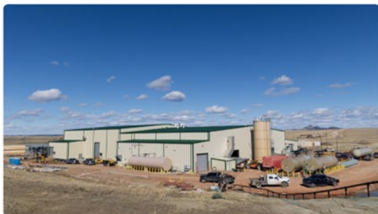
Central Processing Plant (Phase I & II)
