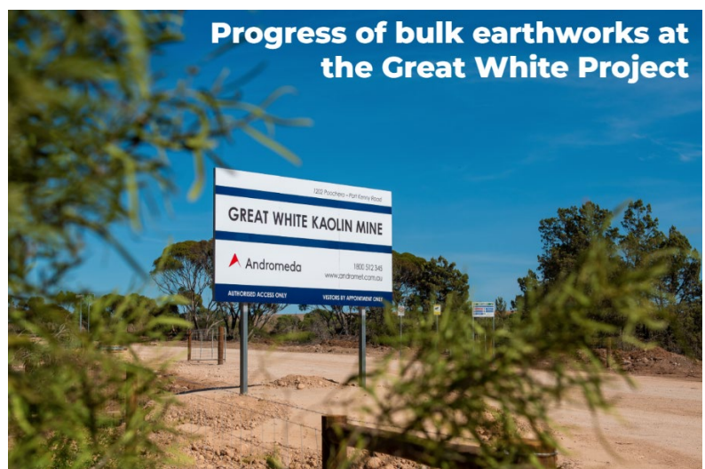
Bulk earthworks in progress
