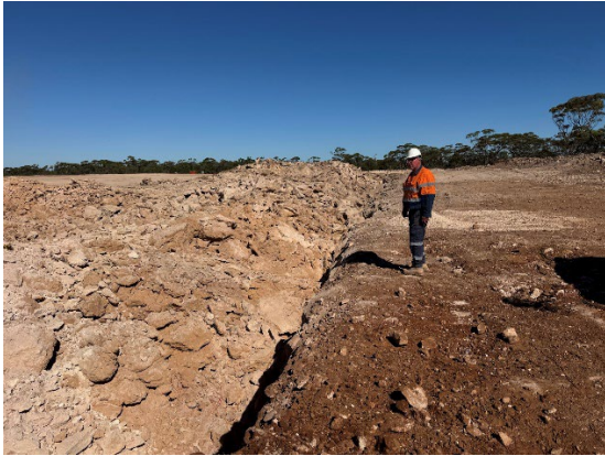
Inspection of blast area following blasting
