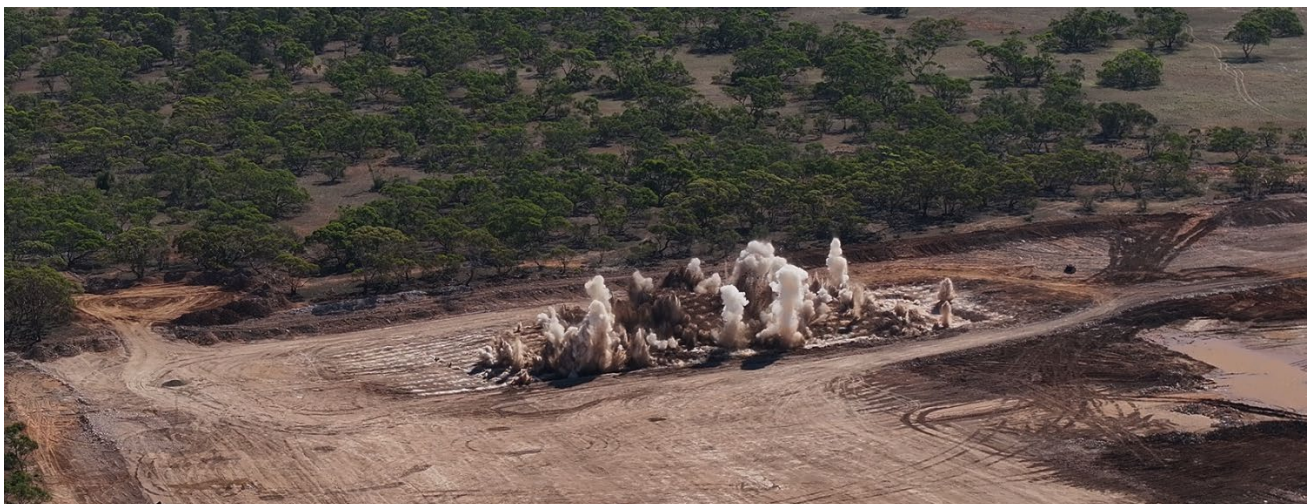
Controlled blasting taking place
