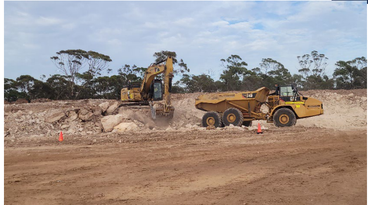
Excavation of blast area following blasting
