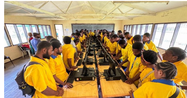
Computers are being installed for a high school in Jiwaka Province as part of the Litehaus International Partnership
