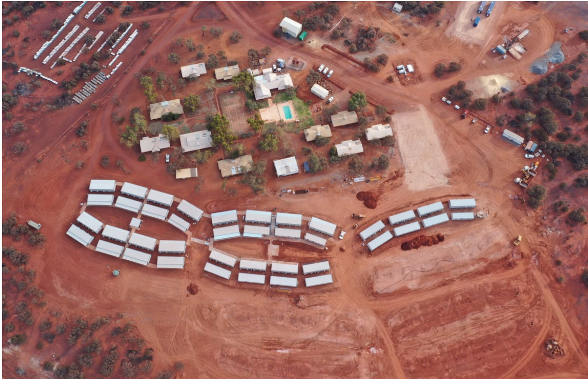
Figure 3 – Camp and expansion works
