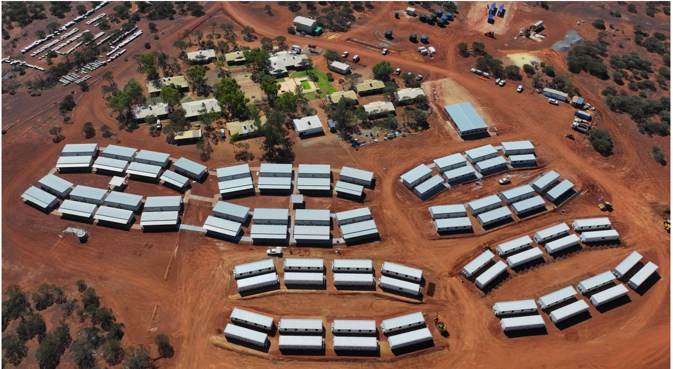
Figure 4 – Camp expansion preparation works advancing
