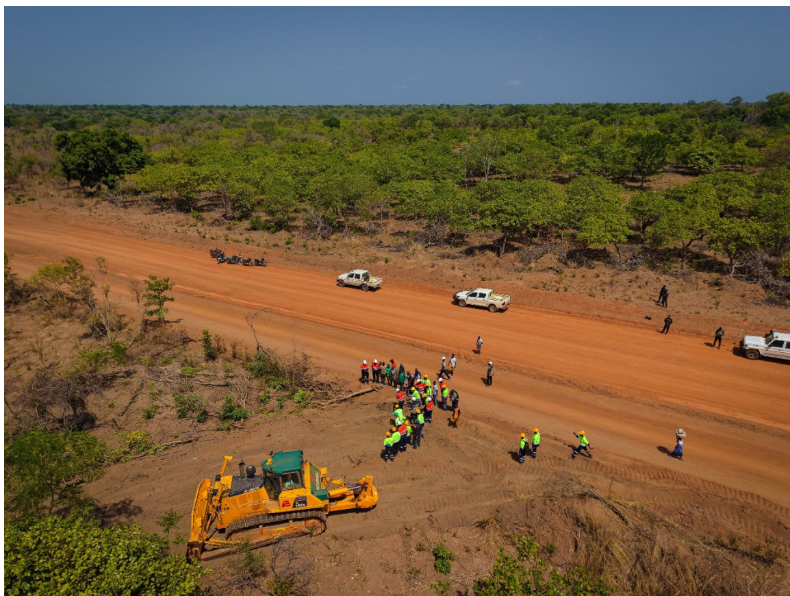
Figure 11: Ground clearance activities
