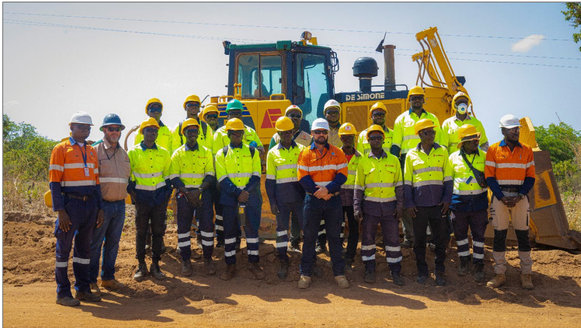
Figure 10: Groundbreaking starting on site
