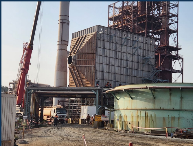
Top Right: Flotation Circuit construction complete and due for commissioning
