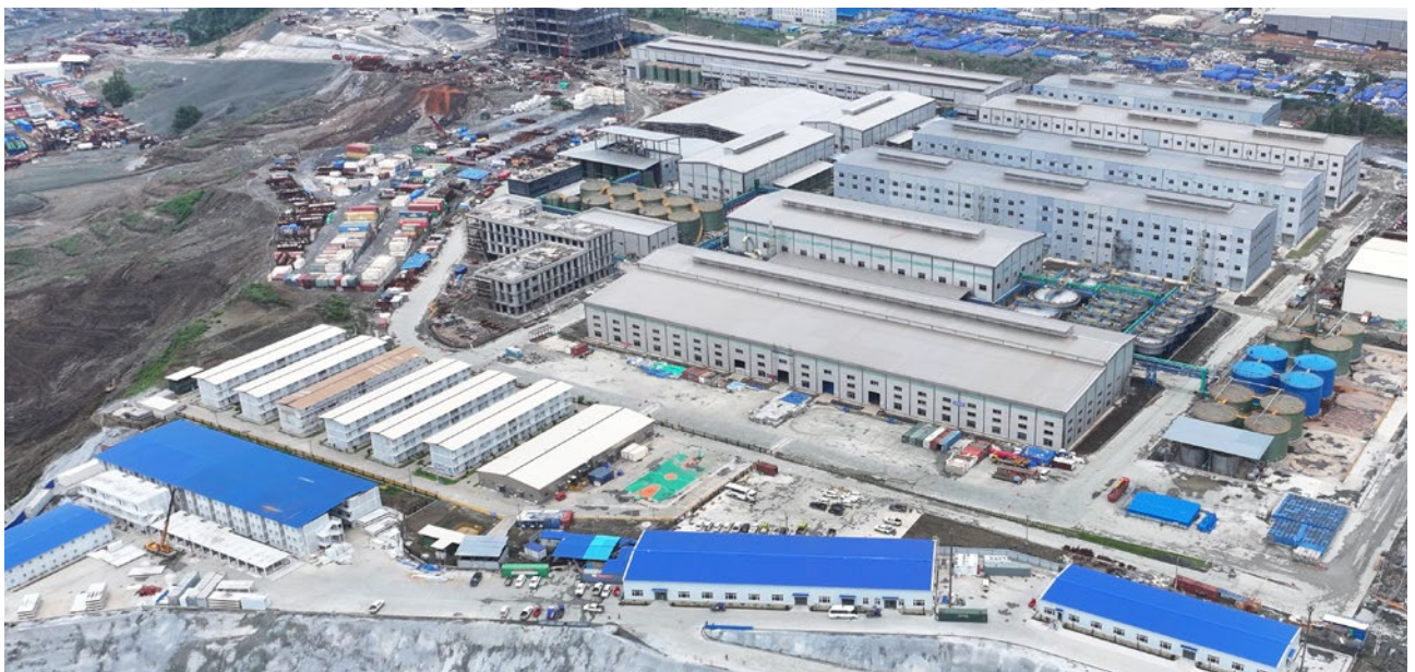
ENC integrated sulfate and cathode refinery construction progress
